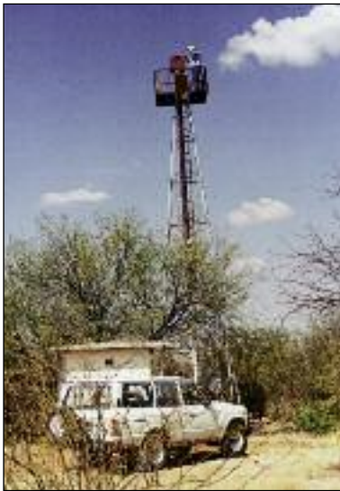
Water level recorder near Stampriet high above ground measuring the artesian water level
