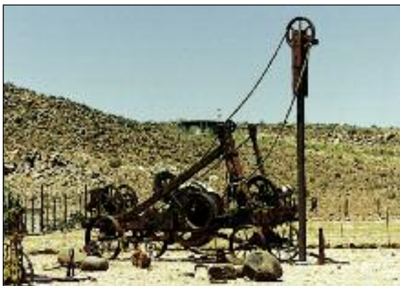
Old drilling machine for groundwater boreholes
